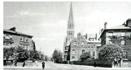
John Loughborough Pearson, St Augustine's Kilburn (1870-7). The orphanage in the foreground has since been demolished.
