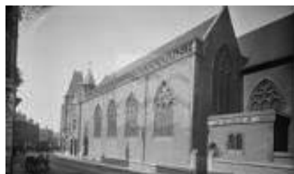
Henry Taunt's photograph of St George's Chapel, George Street, Oxford in 1907. The Old Fire Station (H.W. Moore, 1894) can be seen beyond it.
