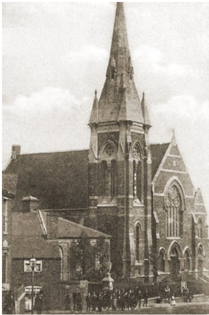
Park Lane Methodist Church, Tipton. George Bidlake (1865, demolished 1975)
