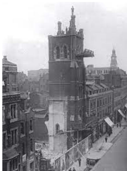
St Jude’s Commercial Street being demolished (1927)
